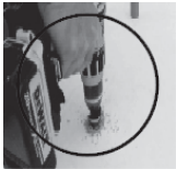
Option C: Drill a hole with a hole saw bit.
